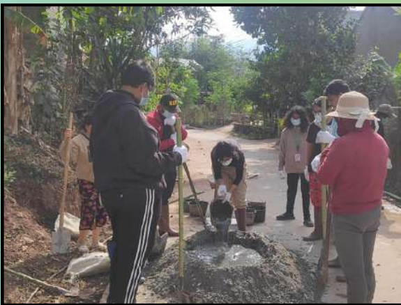
Mixing cement concrete
